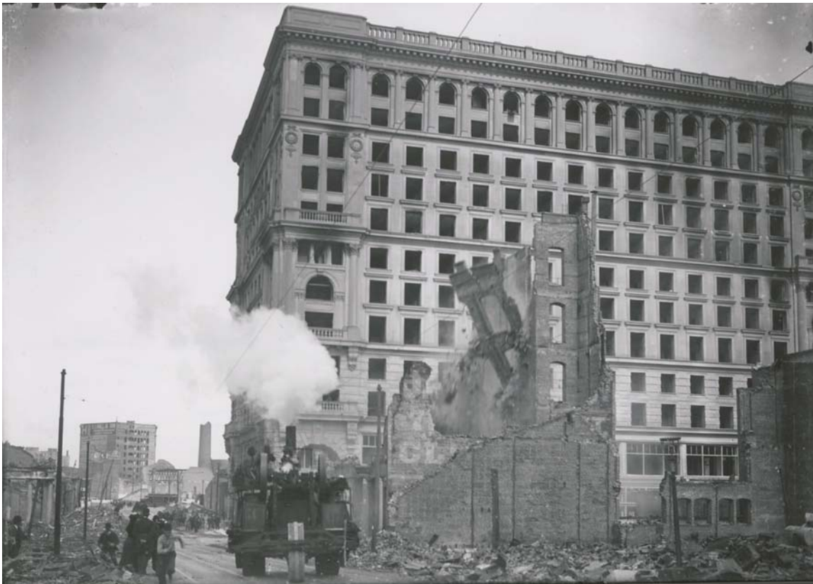
The traction locomotive leased by the Board of Public Works tears down the remains of the Auzerais Building on the southwest corner of Ellis and Powell. California Historical Society, FN-33837.
