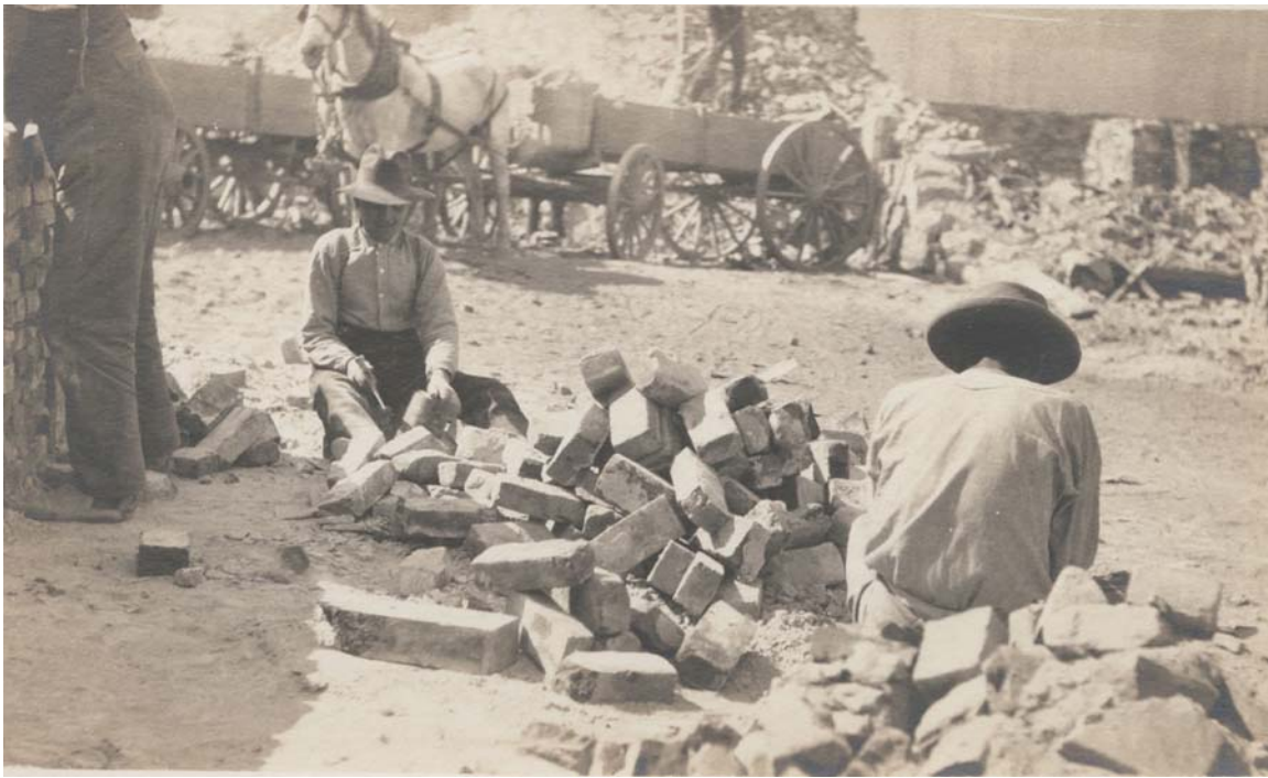
Brick cleaners with hatchets chip mortar off bricks which are then stacked for removal or reuse. In the background wagons are being loaded with rubble. California Historical Society, FN-33928.
