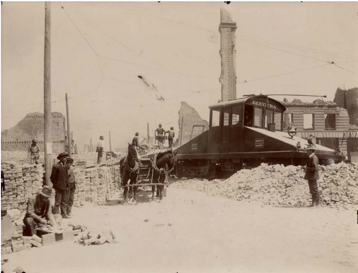
Electra at Battery and Market. The basic elements of debris clearing are depicted here: the brick cleaner with his hatchet; men pushing wheelbarrows of rubble up a plank to dump into a debris car; cleaned bricks stacked; a team ready to haul bricks or rubble. California Historical Society, FN-33849.
