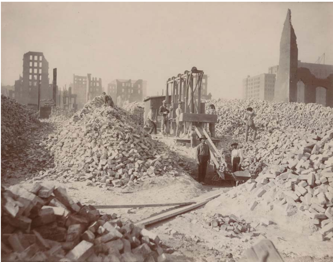
“Patent cleaner at work in a debris brick mine” proclaimed the caption on this photograph when it appeared in Sunset for October, 1906. Bricks may have been brought to this site, near Ellis and Mason, for rapid cleaning. Powered grinding wheels made short work of mortar adhering to brick. California Historical Society, FN-12385.
