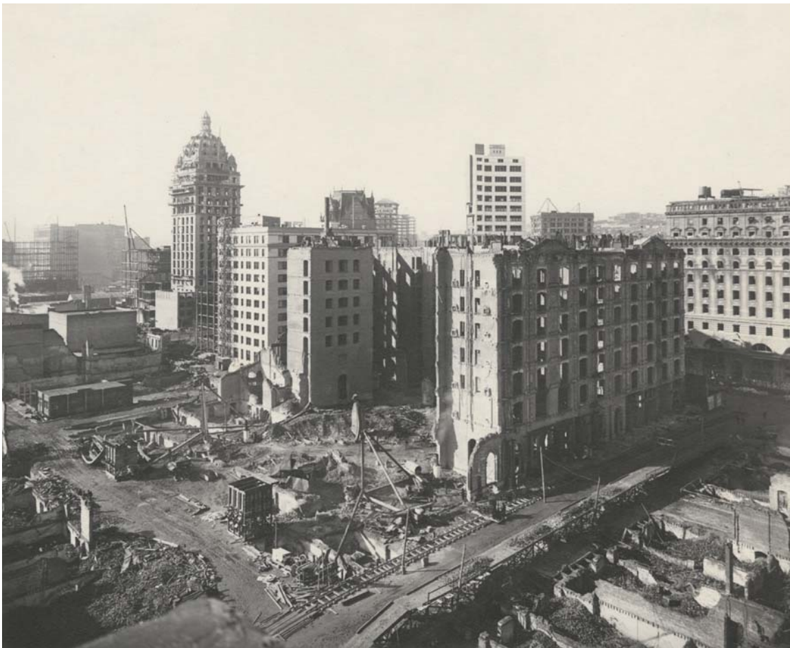
The New Montgomery bunker. Wagons dump their loads on the bunker platform, and the rubble is shoveled onto flatcars waiting below. Originally the bunker possessed two platforms. Track next to the Palace Hotel will carry flatcars full of crushed brick. The machinery is being assembled at the corner of Jessie and New Montgomery. Note the two debris bunkers for loading wagons. California Historical Society, FN-18759.
